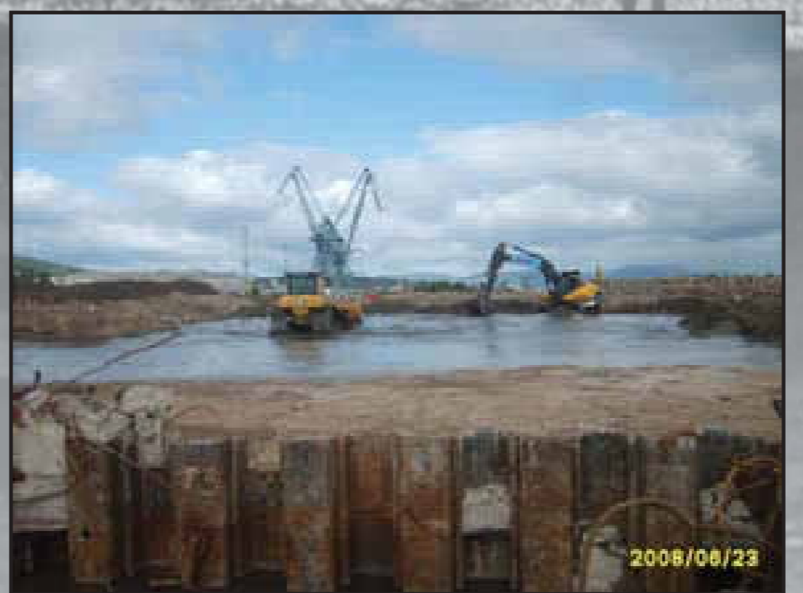
Earthworks within the central section of the basin
