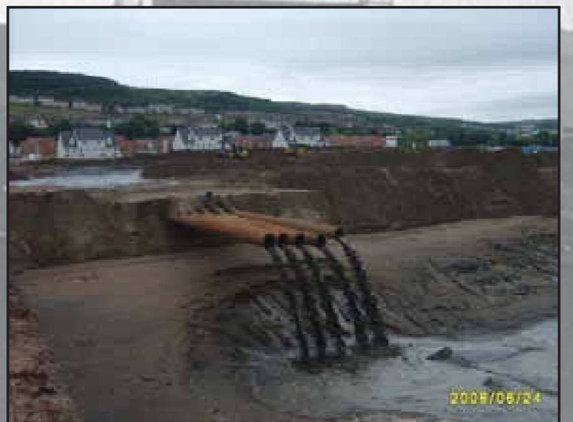
Pipes used for draining the water
