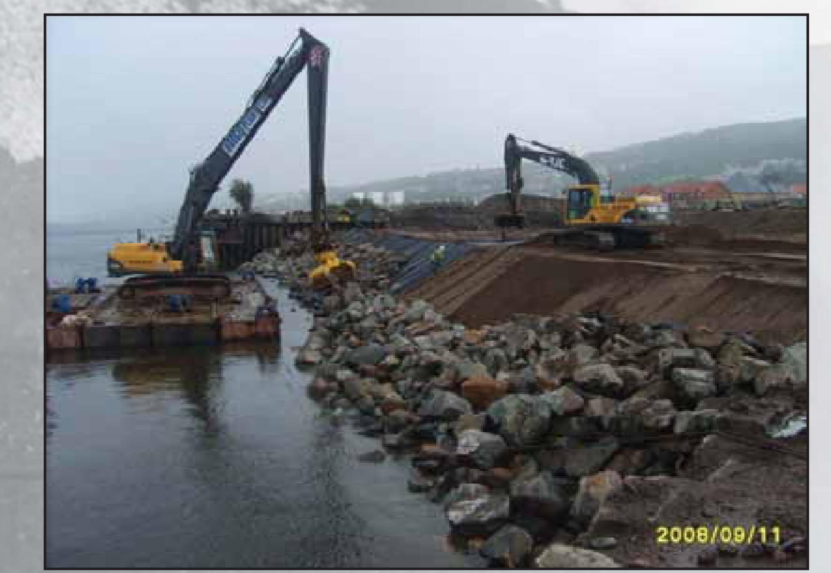
Placement of rock armour erosion protection on the face of the Basin Closure Bund
