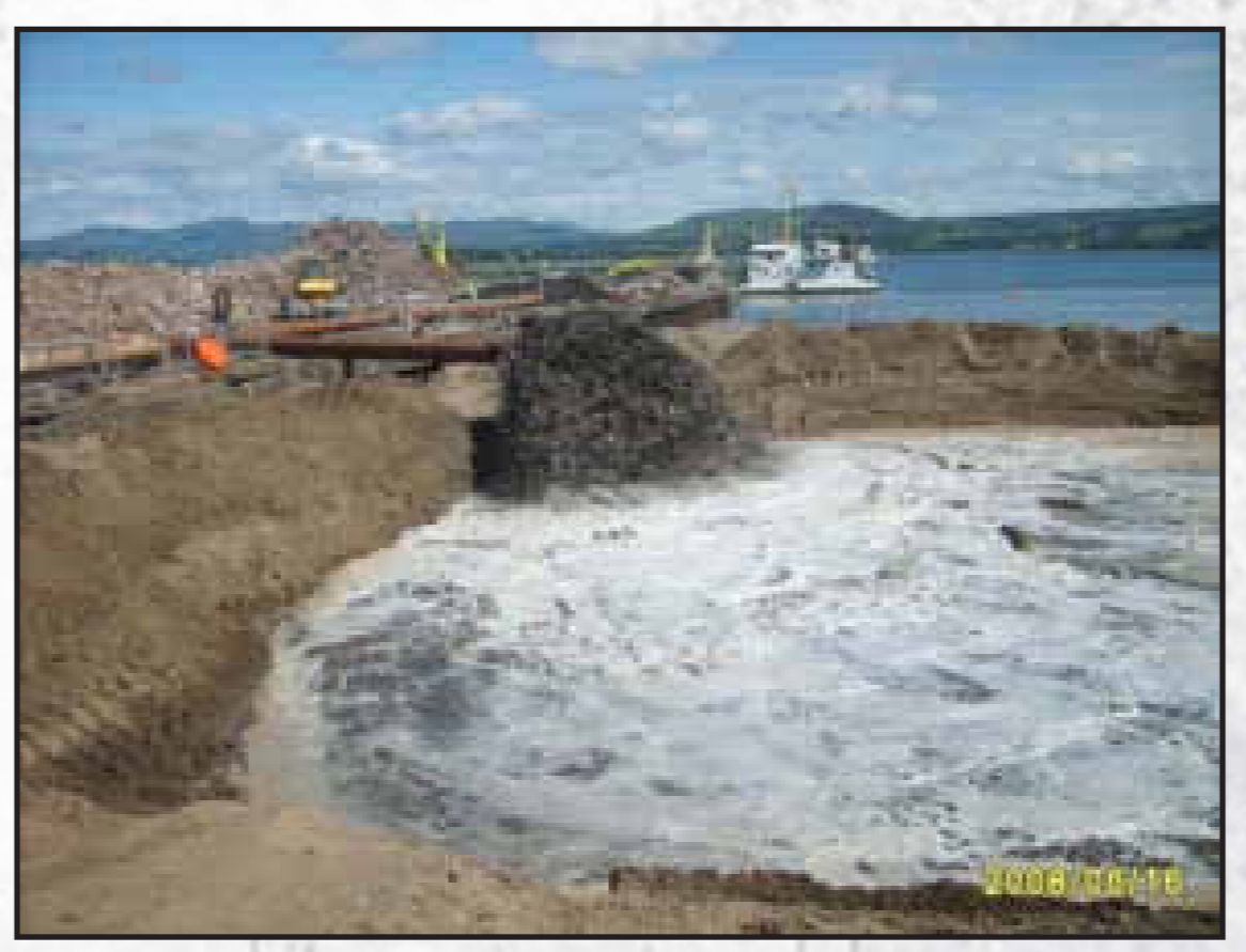
Sand/water mix being pumped into one of the sections of the basin (the dredger is visible in the background)
