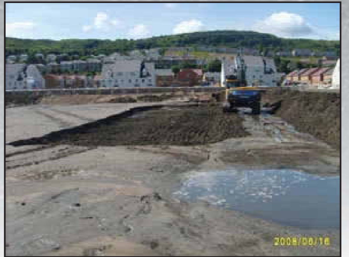
Removal of excess sand to create sufficient space to allow the next load of dredged sand to be delivered
