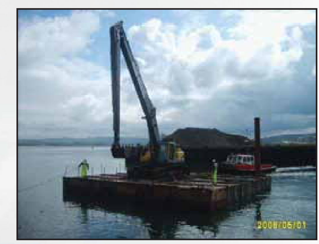
Placement of rock armour erosion protection on the face of the Basin Closure Bund
