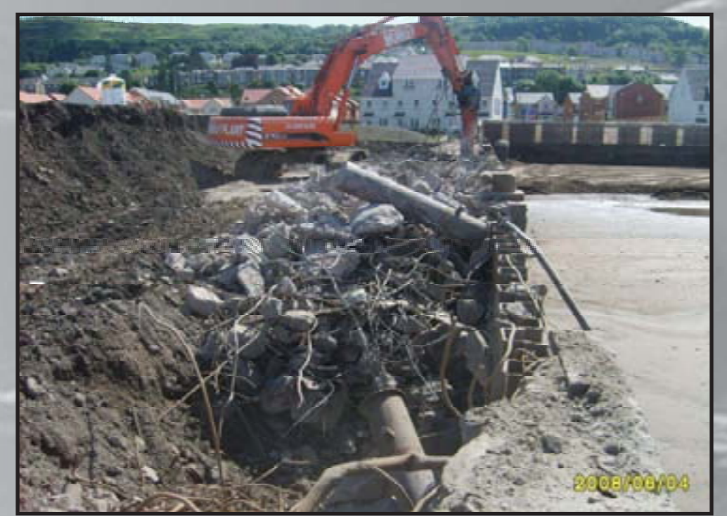
Breaking out of heavily reinforced structures adjacent to the dock
