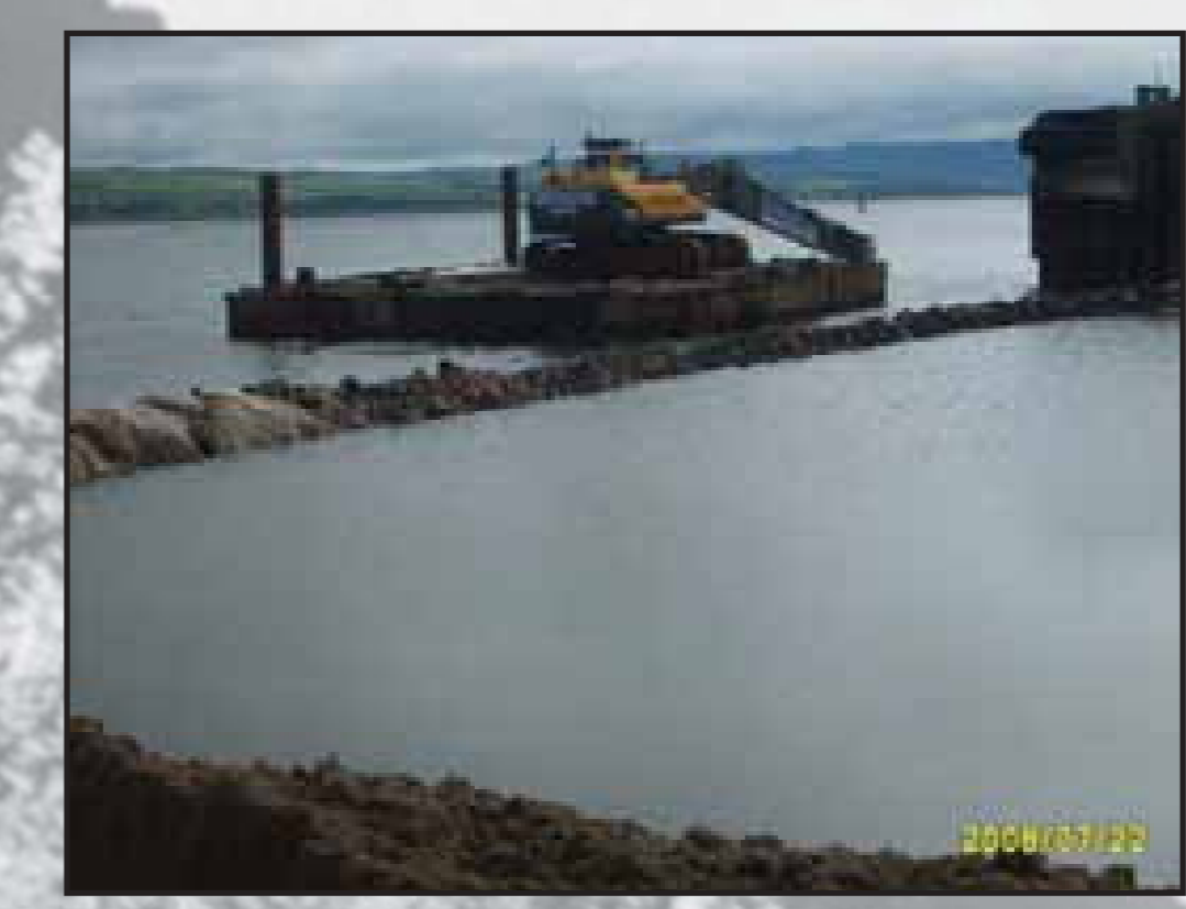
Placement of rock armour erosion protection on the face of the Basin Closure Bund
