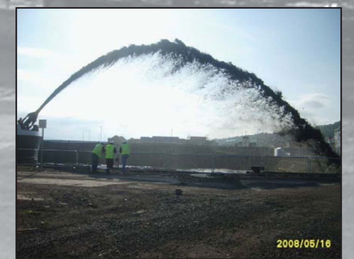
Infilling of the first section (south) of the basin
